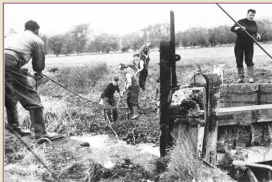
1951. A Volunteer working party on upstream clearance before installing the stank
